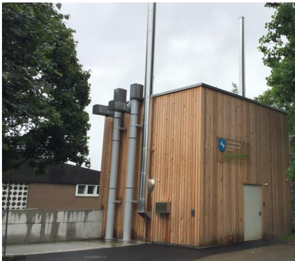
Figure 13.32 Central heating plant as prefabricated element with integrated or additional fuel storage tanks (source: Holzenergie Schweiz).
