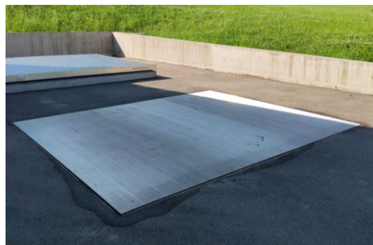
Figure 6.9 Silo lid not accessible in the background and accessible in the foreground. Both in closed condition. (Source: Schmid energy solutions).
