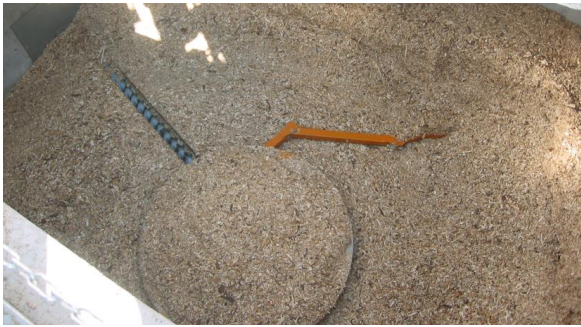
Figure 6.27 Discharge system with articulated arm for quality wood chips and pellets (source: Holz-energie Schweiz).
