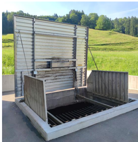
Figure 6.8 Silo lid not accessible when open (source: Schmid energy solutions).
