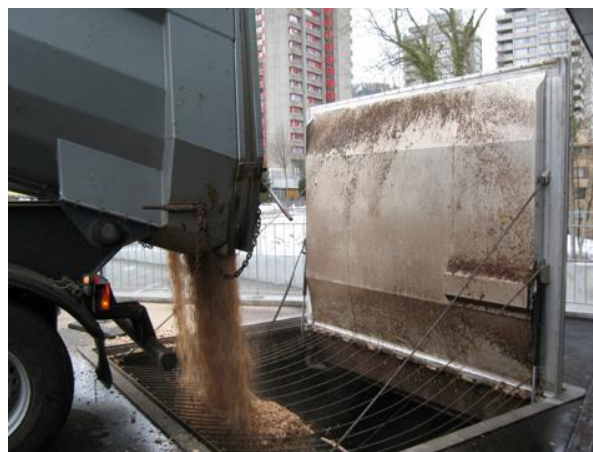
Figure 14.1 Feeding the underfloor silo (source Holzenergie Schweiz).
