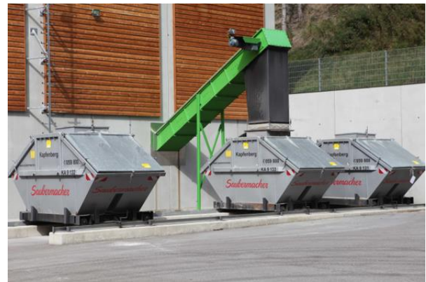
Figure 14.7 Ash trough changing device (source: AEE INTEC).
